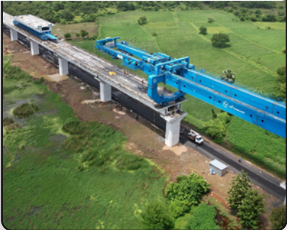
High Speed Rail, Mumbai - Ahmedabad
