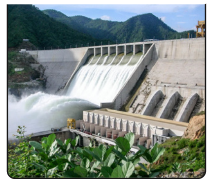
Hydro Power Plant, Bhivpuri
