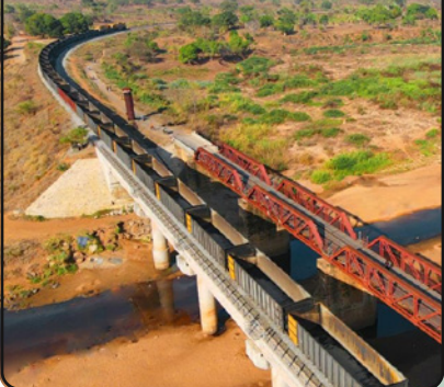
Monapo Bridge, Malawi
