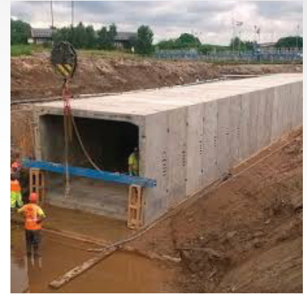
Structural Design for precast boxes
