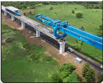
High Speed Rail, Mumbai - Ahmedabad
