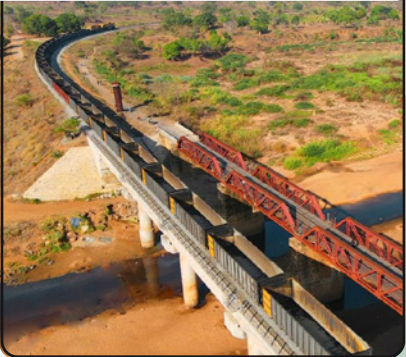
Monapo Bridge, Malawi
