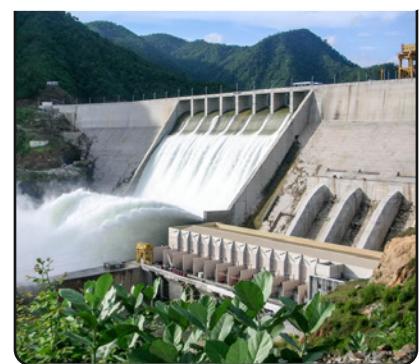
Hydro Power Plant, Bhivpuri
