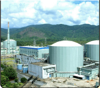
Nuclear Power Plant, Kaiga
